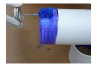
Use primer along with cement, which will allow slightly longer working times. Work quickly to assemble pipe and fitting immediately after solvent cement is applied and still wet.
