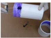
Store solvent cements and primers in a cool or shaded area prior to use. Make sure that both pipe and fittings have been sufficiently exposed to the same ambient temperature. Assemble pipe and fittings in shade if possible.
